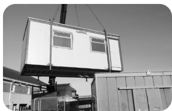
The Westside Community Garden portacabin being lifted into place
